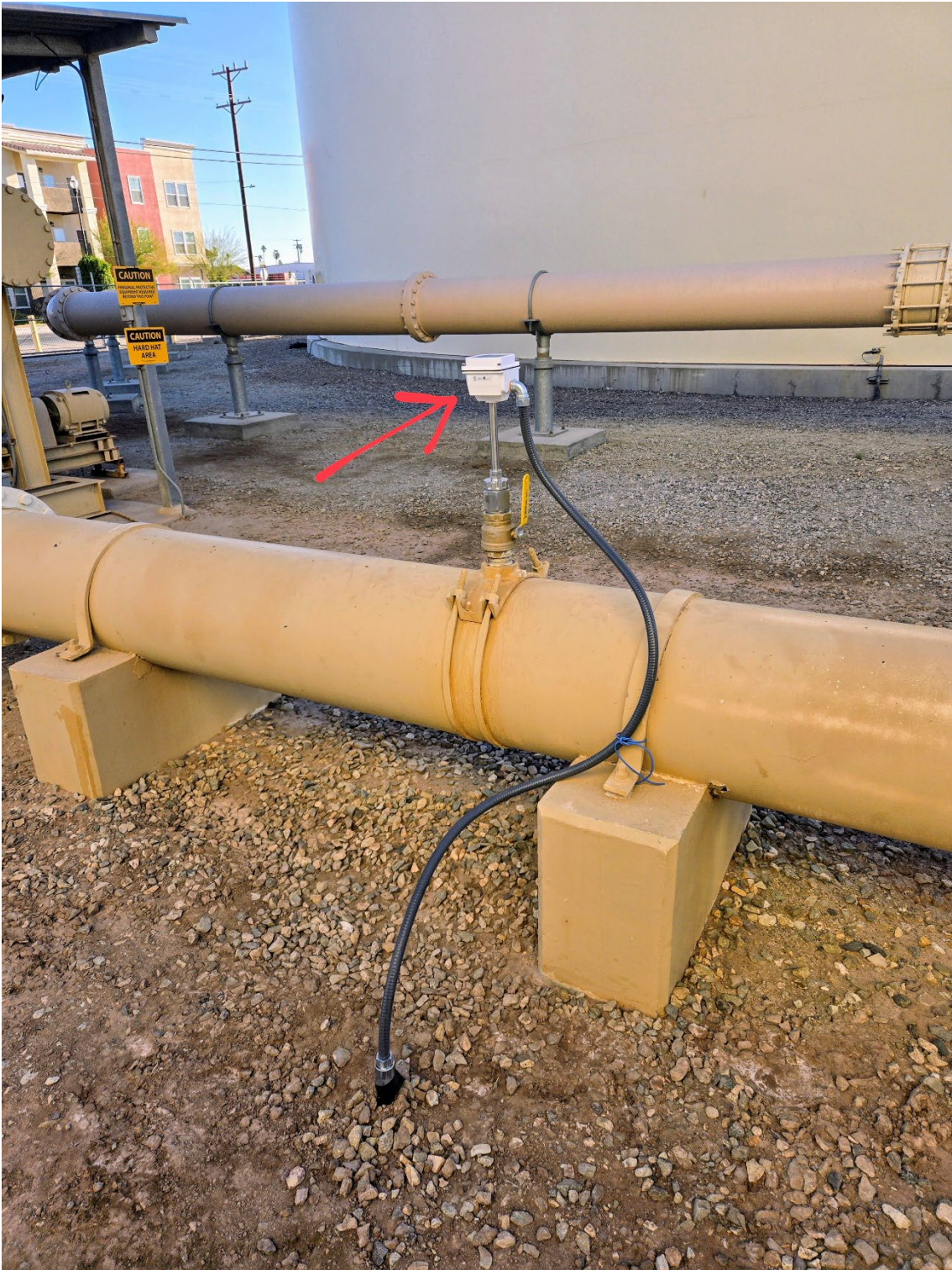
New Seametrics 2" insertion flow meter installation point
