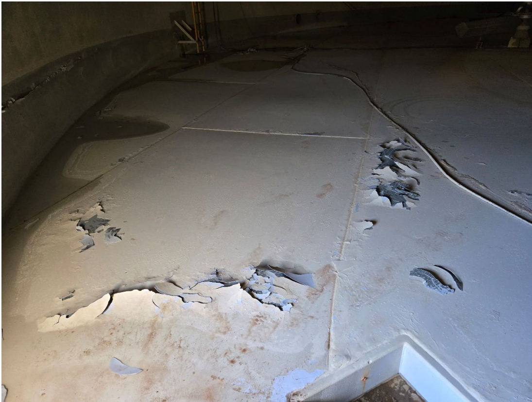
Interior view of drain sump near the bottom access hatch
