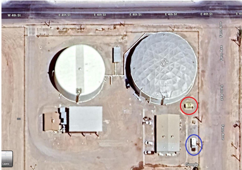
Old water plant gen-set site circled in RED New main gen-set circled in BLUE
