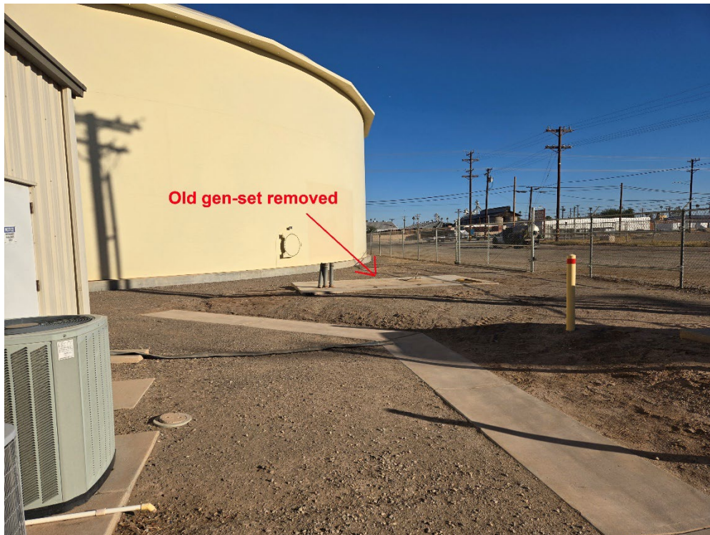
Old gen-set removed from concrete slab foundation
