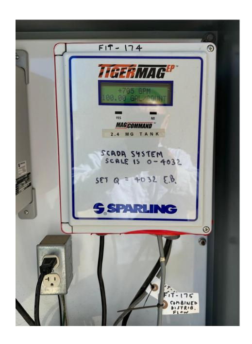
2.4 MG Tank Sparling TigerMag flow transmitter.
